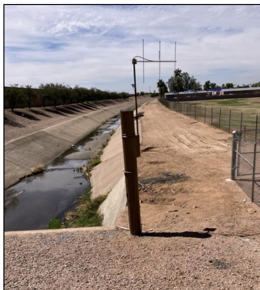
'Skyline Park' Rain Gage, Station No. 50902, Installed 12/05/2024
