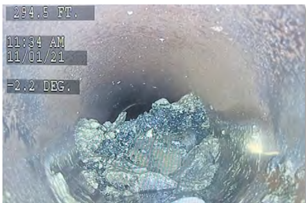
Sewer main before hydro cleaning:
