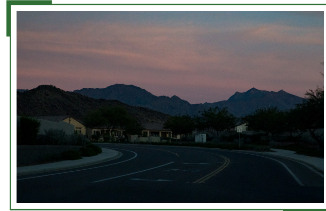
Minor collectors serve an important role in connecting neighborhoods to the arterial roadway network.
