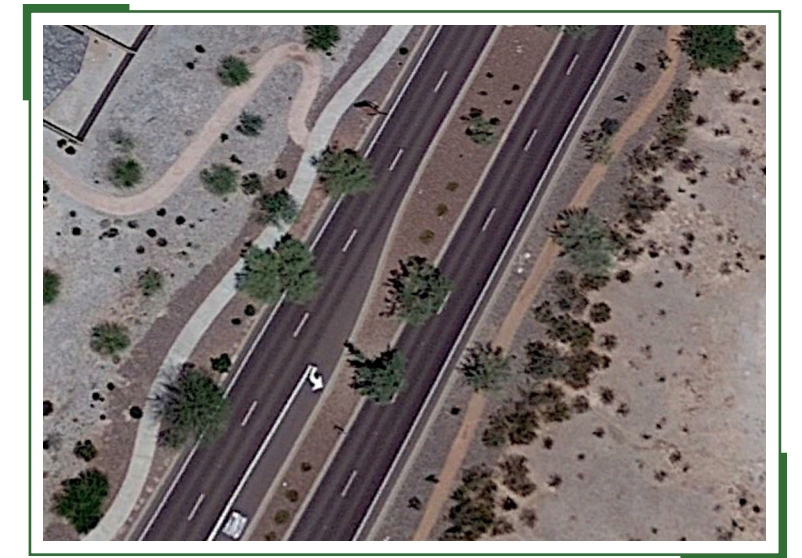
Estrella Parkway is a Scenic Arterial, and ultimately envisioned to be three travel lanes north and south throughout Goodyear with bicycle lanes and sidewalks.
