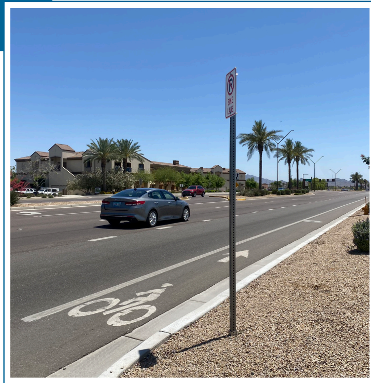
Goodyear's street standards call for bicycle lanes on all arterial and collector streets.
