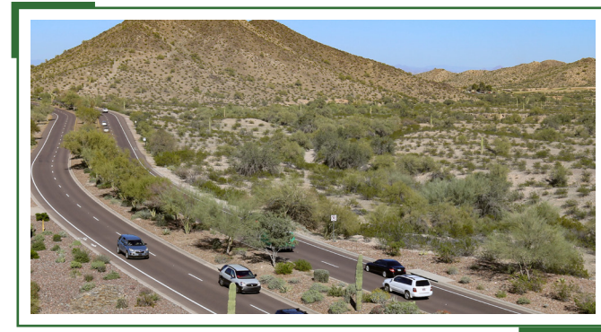
Pebble Creek Parkway and Estrella Parkway (pictured here) is a Scenic Arterial stretching north to south across Goodyear.
