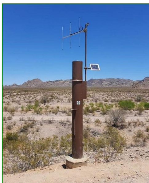
'Middle Harquahala FRS' Rain Gage, Station No. 50258, Installed 05/18/2022
