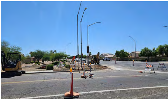
Northern Traffic Signal construction at 111 th Avenue
