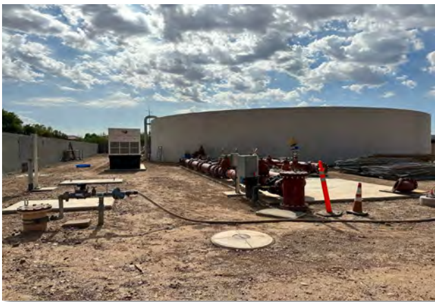
Salter Well Site Rehabilitation
