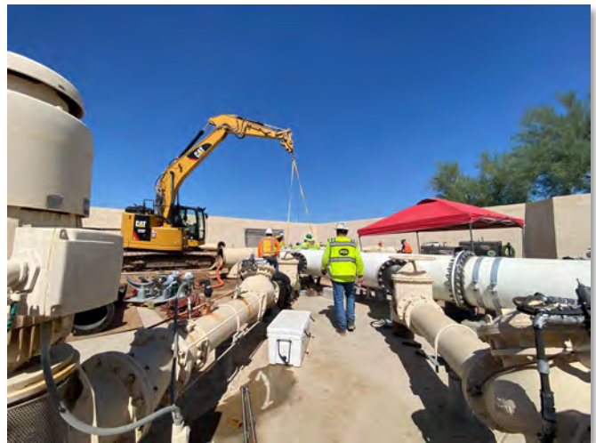
Jomax Booster Pump Station Upgrades
