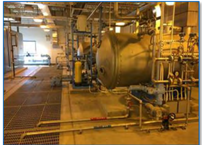
Greenway Water Treatment Plant
