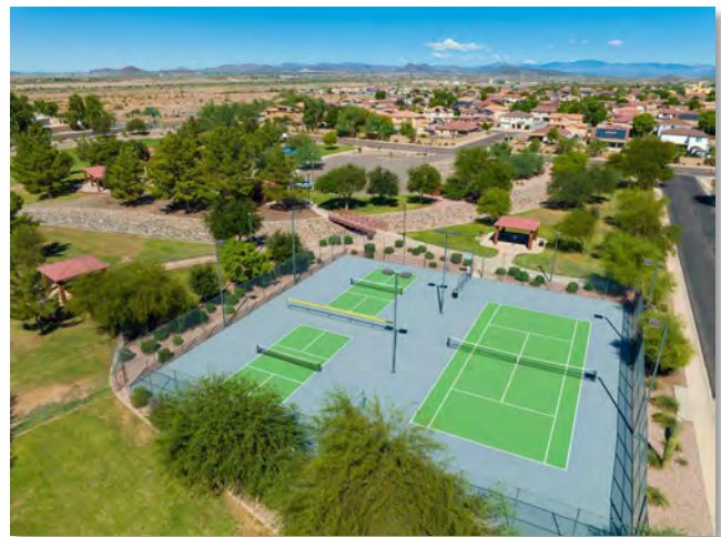
Alta Vista Tennis Court Renovation
