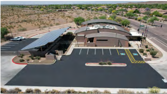
Fire Station 196 on El Mirage Road Facility Parking Lot Improvements
