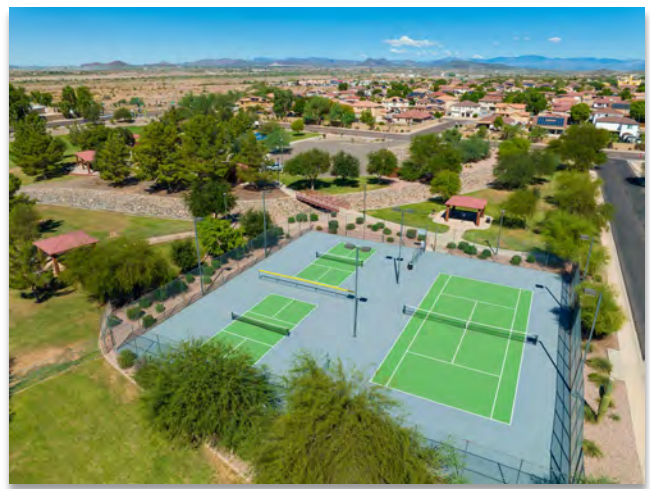
Alta Vista Tennis Court Renovation
