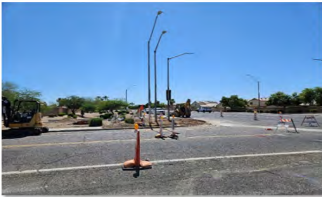
Northern Traffic Signal construction at 111 th Avenue
