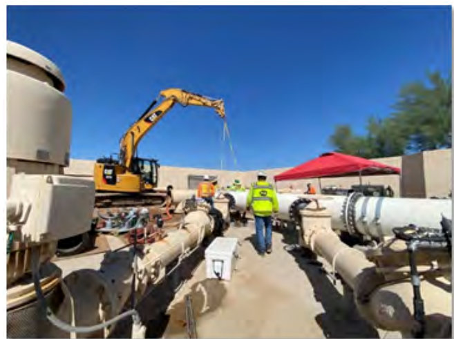
Jomax Booster Pump Station Upgrades
