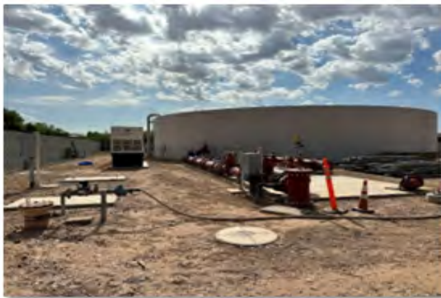
Salter Well Site Renovation
