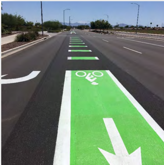
Green bike lanes provide visible and designated areas for bicyclists to share Peoria’s roadways
