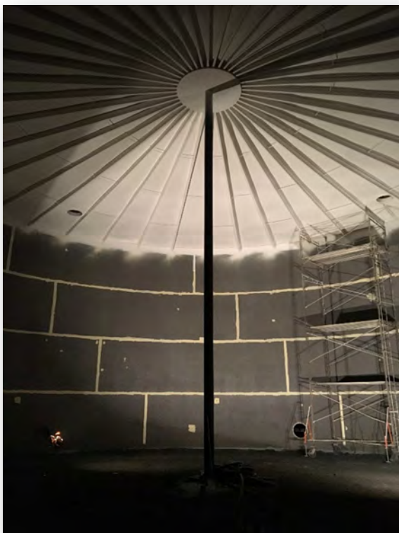
The inside of the Arrowhead Shores water reservoir during its rehabilitation
