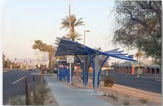
Shade sails along Peoria Avenue were funded by way of the Transportation Sales Tax
