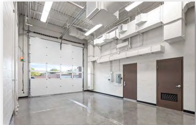
Fire Station No. 2 Dorm Expansion included additional space for a vehicle bay
