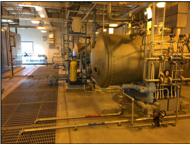
Greenway Water Treatment Plant
