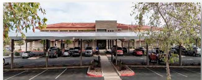
Solar Panel Parking Canopy at the Development & Community Services Building
