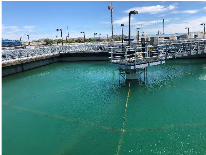
Greenway Water Treatment Plant Basin Cleaning
