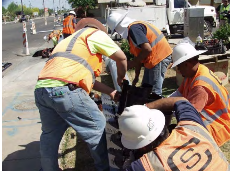
Traffic Signal Repair at 91 st Avenue and Northern
