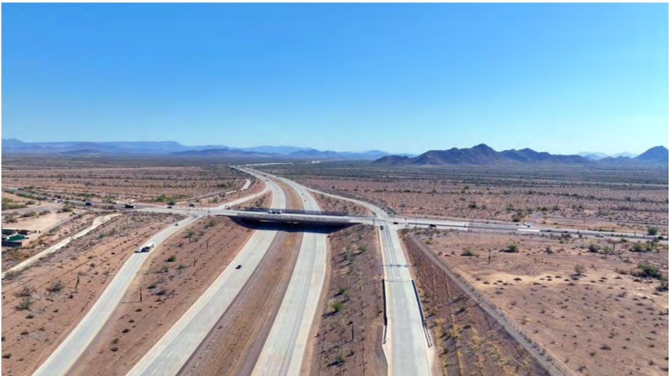
Lake Pleasant Parkway Overpass on Loop 303
