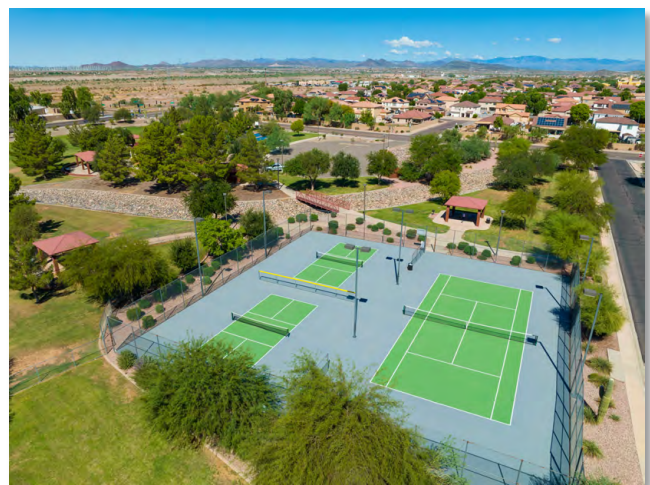
Alta Vista Tennis Court Renovation
