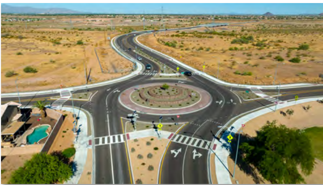
Deer Valley roundabout connection at 109 th Avenue
