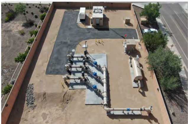
Sonoran Mountain Ranch Booster Station Rehabilitation
