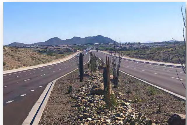
The newly widened Happy Valley Parkway from Loop 303 to Lake Pleasant Parkway
