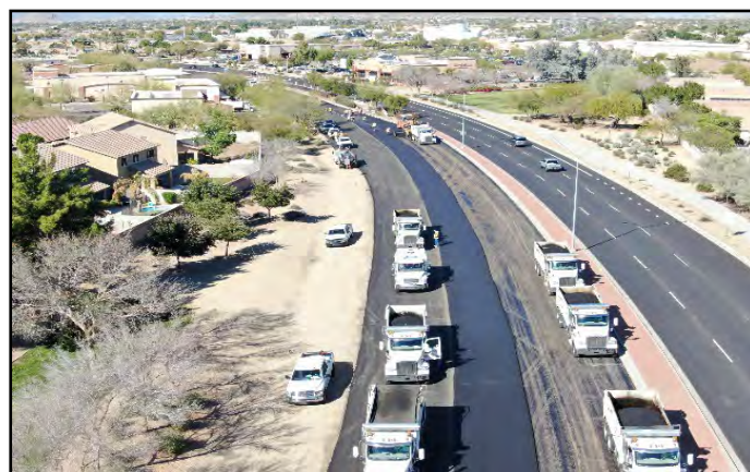
Street maintenance crews repaving Peoria roadways
