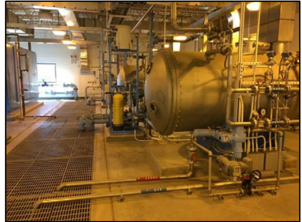
Greenway Water Treatment Plant
