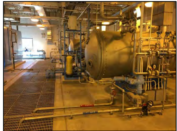
Greenway Water Treatment Plant
