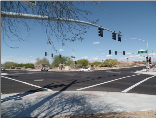
Deer Valley Road Improvements
