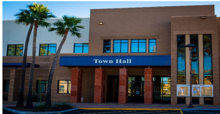
Fountain Hills Town Hall
