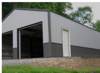
WRF Equipment Building
