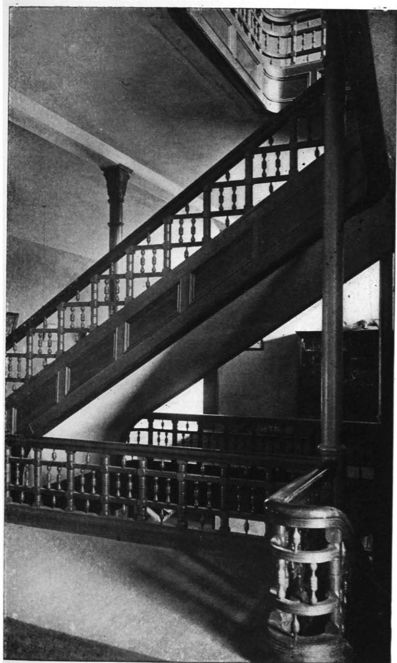
STAIRWAY IN MAIN BUILDING
