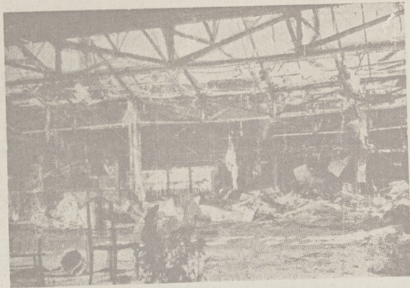
Shanghai North Station
