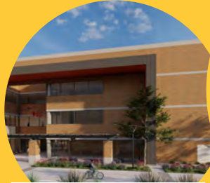
New academic building, occupancy in spring 2025.
