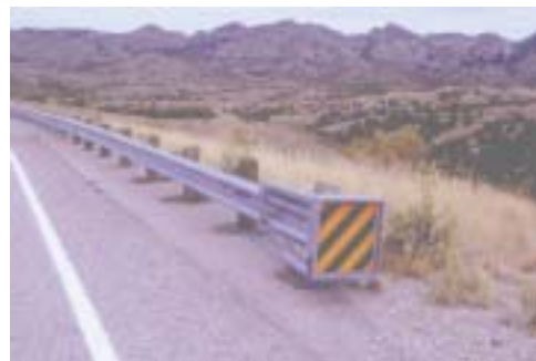
Existing guardrail along the Scenic Road
